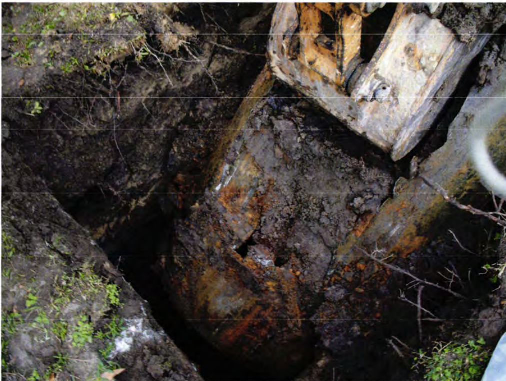
Picture 2: UST 440Elderberry being removed from the excavation.
